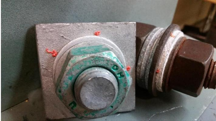
DuraSquirt® DTIs, are enhanced ASTM F9591 DTIs that render feeler gauges unnecessary. Like Squirter® DTIs, DuraSquirt® DTIs expel orange indication media when a bolt has been properly pretensioned in accordance with AISC/RCSC specifications. The difference with DuraSquirt® DTIs, is the indication media is permanent, unless actively removed.
