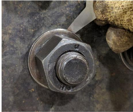
Standard DTIs to be installed and inspected using Feeler Gauge only.
