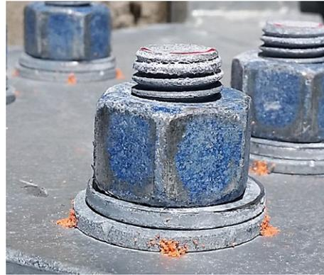
Squirter® DTIs may be installed visually but visual inspection will depend on environmental condition and elapsed time between installation and inspection. If indication media falls away, feeler gages must be employed for inspection purposes.
