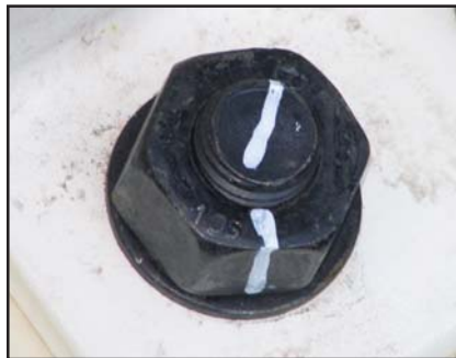
Can you tell how much turn was put on this bolt?
