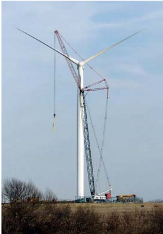
(see figure 1 here – Typical Generator)
