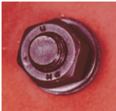
2. Before tightening, there is no red showing around the bolt.
