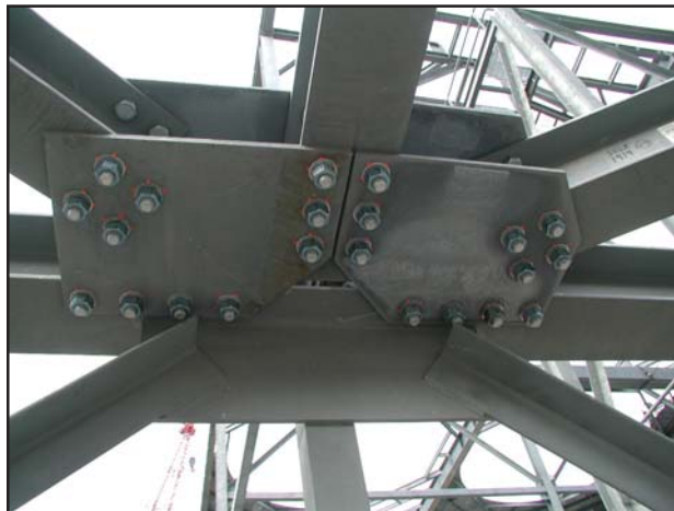
Figure 1: Squirter DTIs came out of construction concerns
