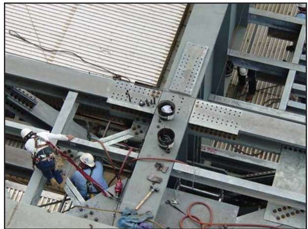
Figure 5: Power plants use hundreds of thousands 1-1/8” A490 Bolts
